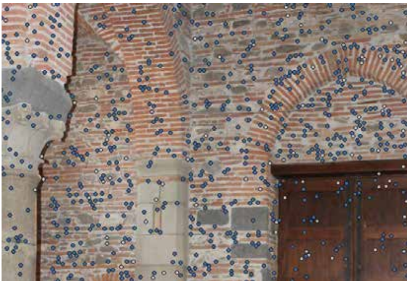
Fig. 3. Image correspondences, or tie points, detected on a church interior photo.
